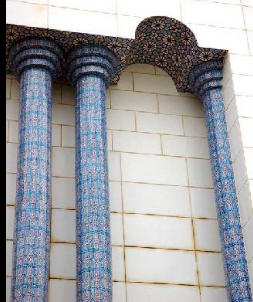
King Fahd Mosque, Culver City
