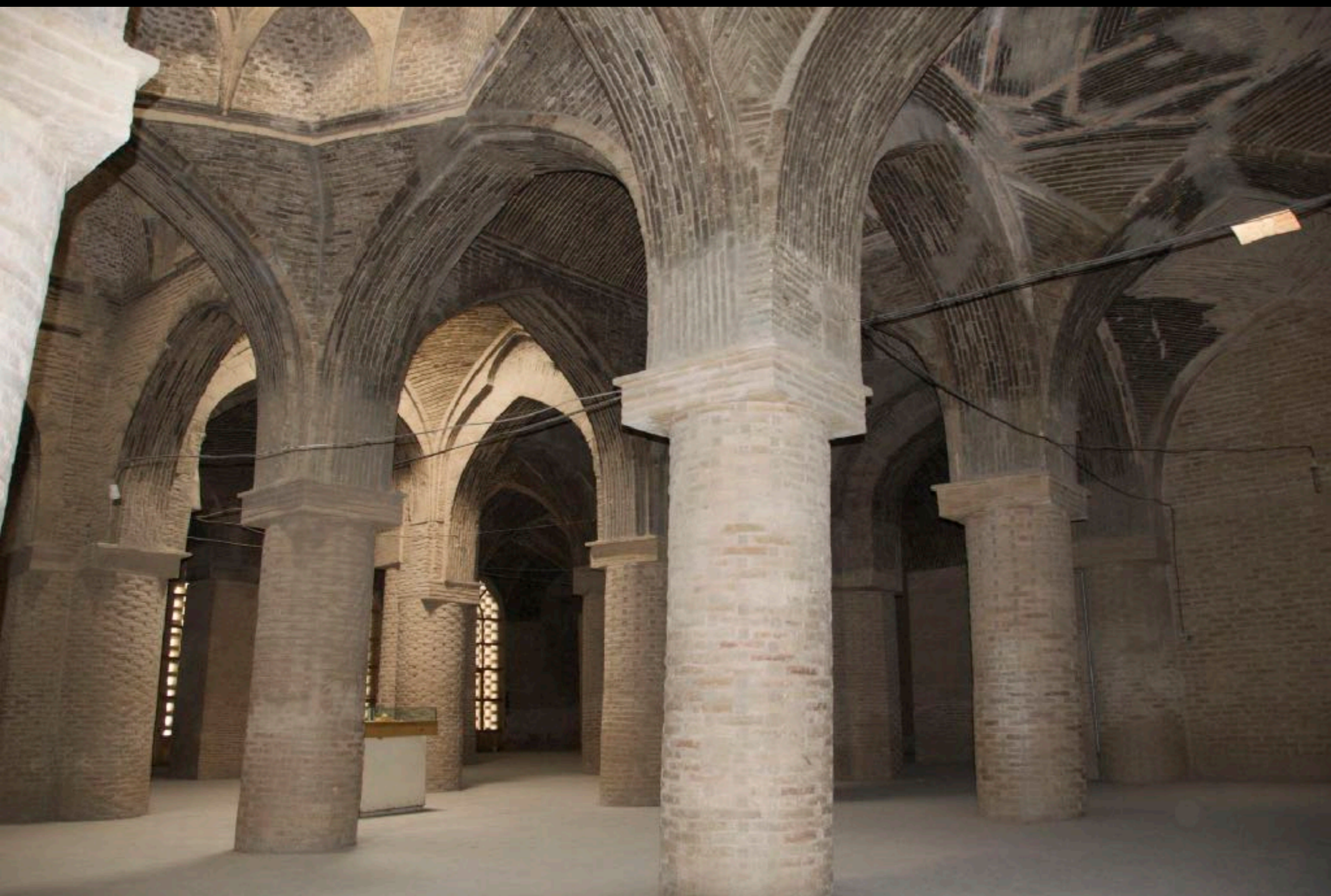
Congregational Mosque, Isfahan (central Iran). Founded Late 8th century; major additions/expansions in 12th century (Saljuq) and onward. Madrasa on southeast.
